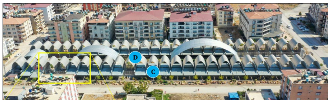
Figure 2: Key aspects of the Centre design, with reference to earthquake resistance. Aerial images courtesy of the Taiwan-Reyhanlı Centre for World Citizens.
